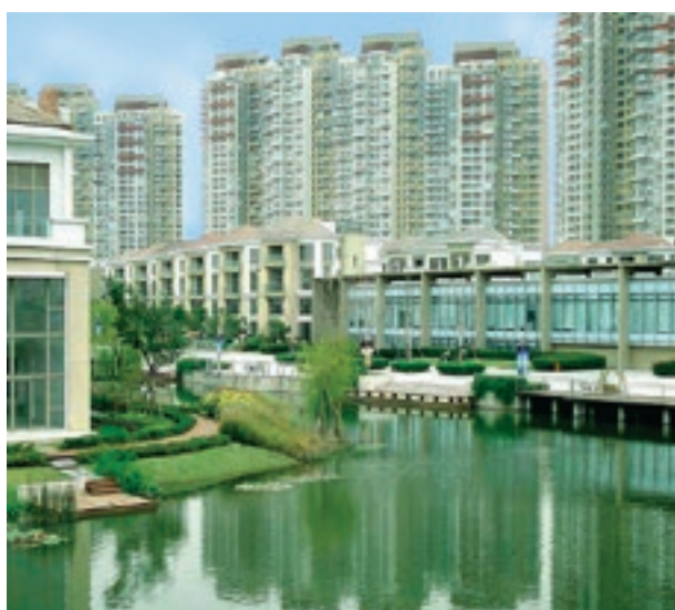
Landlord Butterfly compound, Kunshan
