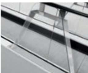
Anti-climb barrier (EN115-1:2008 + A1:2010 requirement)
