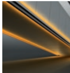
Side and soffit cladding*
